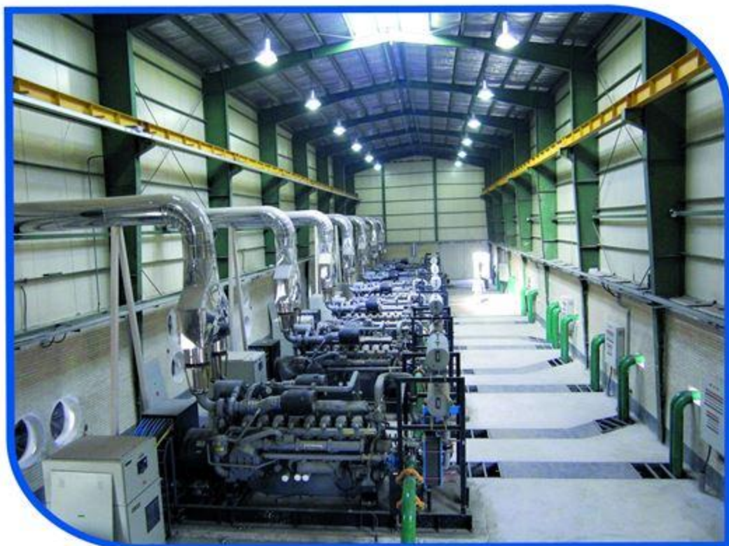
16-MW power plant project in Yazd
